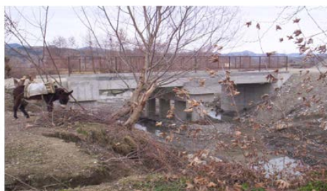
New Bridge in Kocaj, Baldushk
